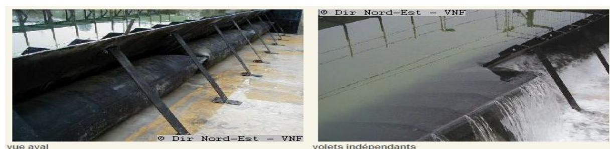
Figure 18: Barrages gonflables
