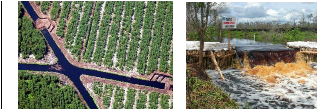
Figure 1 Water management technology: comb structures applied to HTI drainage channel at Kampar Peninsula, Riau (left) and Tabat (right) applied to agriculture land rehabilitation in central Kalimantan
