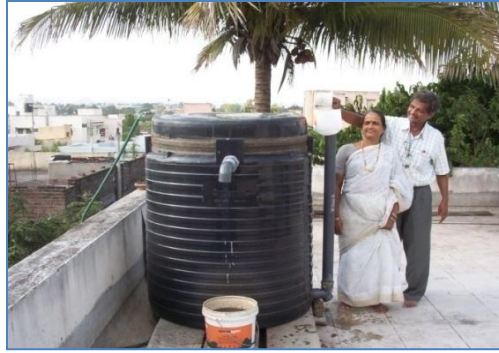
Figure 1– ARTI Biogas Reactor
