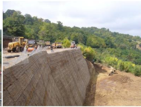
Fig 2. 'Terramesh' method used for Bodbe landslide
